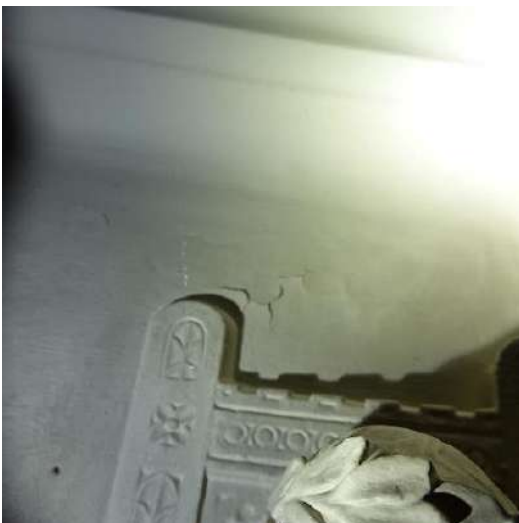
Opstuwing overschildering
